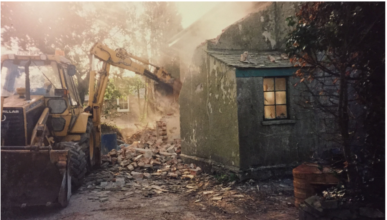
The start of the renovations in 2004
