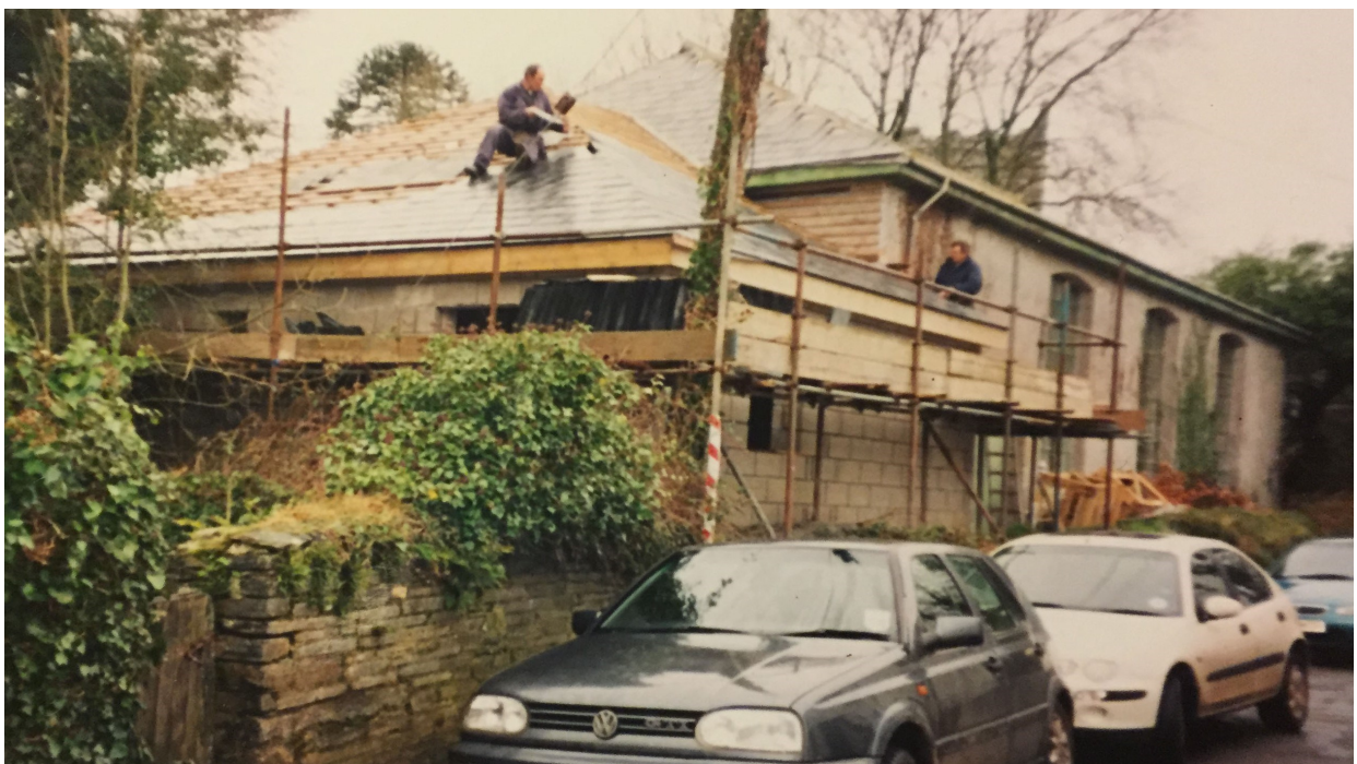
Photos showing the refurbishment of the Church Hall that took place in 2004
